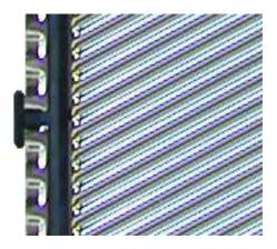
The gasket is double around the ports to prevent intermixing of the two fluids. In the event of gasket failure, any leakage is vented external to the equipment.
